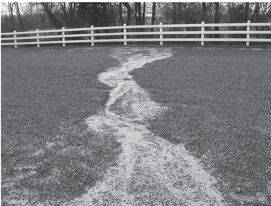
Figure 2. Rubber pieces can float to the top of a footing mixture after large rainfall events. The rubber will have to be mixed back into this stonedust mixture with surface conditioning equipment.
